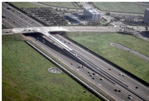
Figure 8: This direct ramp in Los Angeles allows HOVs to enter and leave the median HOV lanes without having to weave across congested general traffic lanes or get caught in delays at a nearby interchange [9].
