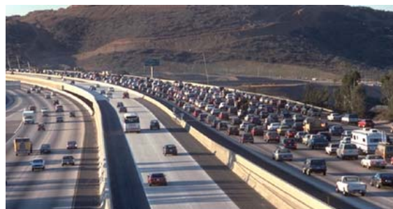
Figure 9: I-15 in San Diego has a 13 kilometre long barrier-separated reversible two-lane core available free for carpoolers and for a price (which varies according to demand and congestion levels) to non-HOV users [10]. Part of the toll revenue is dedicated to enhancing I-15 bus service.
