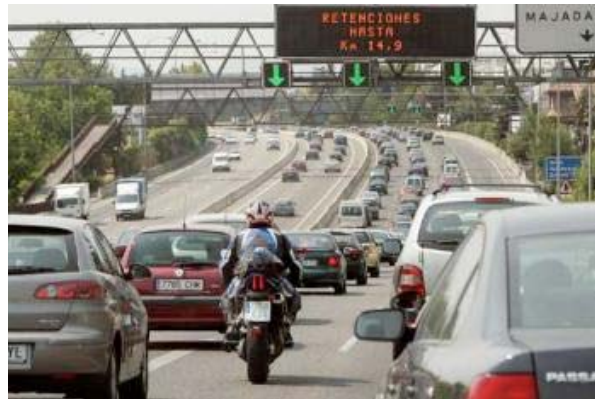
Figure 1: In Spain, Madrid's N-VI median reversible HOV lanes (centre distance of photo) have operated successfully since 1995 [1].
