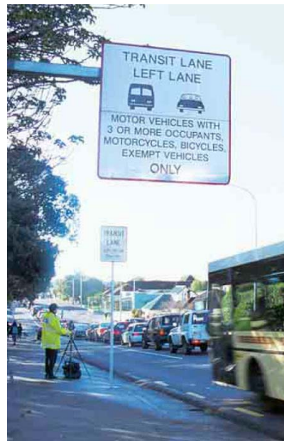
Figure 14: An AM peak period curbside HOV 3+ lane on Onewa Road in Auckland, New Zealand has been in use since 1982. Dramatic improvement in HOV lane operations occurred in 2003 after municipal parking control officers were trained by the police and granted the responsibility of enforcing HOV lane operation. Now new HOV lanes are being planned in the area [15].
