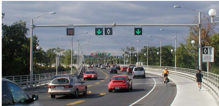
Figure 10: A reversible HOV 2+ lane is used in Ottawa, Canada to maximize the person-carrying capacity of a three-lane bridge crossing [11].
