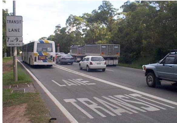
Figure 13: In Brisbane, Australia (as in several U.S. centres), HOVs are provided with bypass lanes at signal-controlled motorway entrance ramps [14].
