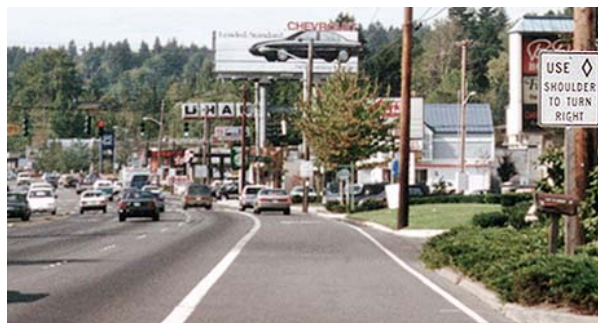
Figure 12: This photo illustrates a right-side HOV 3+ lane in Seattle, US, that can be used by motorists for access to mid-block entrances [13].
