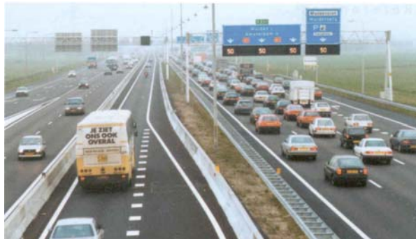
Figure 2: The N4 near Amsterdam was a barrier-separated HOV 3+ facility that operated from 1993 to 1994. It did not attract enough users to overcome public criticism and was opened to general traffic [2].
