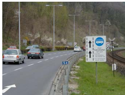
Figure 4: In Linz, Austria, the sign on B127 (opened 1998) notes that “ This (bus) lane can also be used by (1) small cars with minimum 3 passengers and (2) livestock trucks ”[5].
