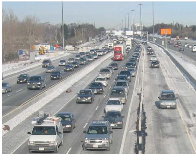
Figure 6: From Toronto, Canada, this photo of Highway 404 illustrates “best practice” for motorway HOV lanes – a painted buffer separator, designated areas for HOV lane access and egress, extensive signage, wide shoulder adjacent to the HOV lane for enforcement purposes, and protected pockets in the median (not shown) for police observation [7].
