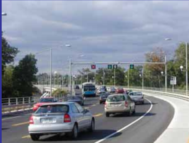
Reversible HOV lane on 3 lane bridge
